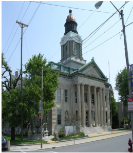
CRAWFORD COUNTY COURTHOUSE
