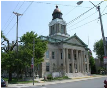
CRAWFORD COUNTY COURTHOUSE
