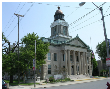
CRAWFORD COUNTY COURTHOUSE
